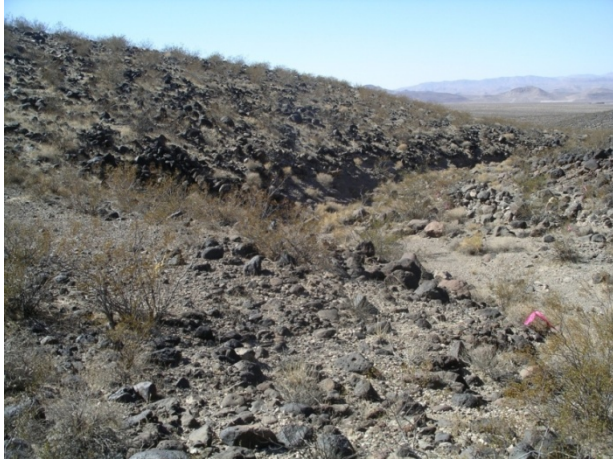
Figure 46. Existing Natural Stormwater Conveyance Channel
